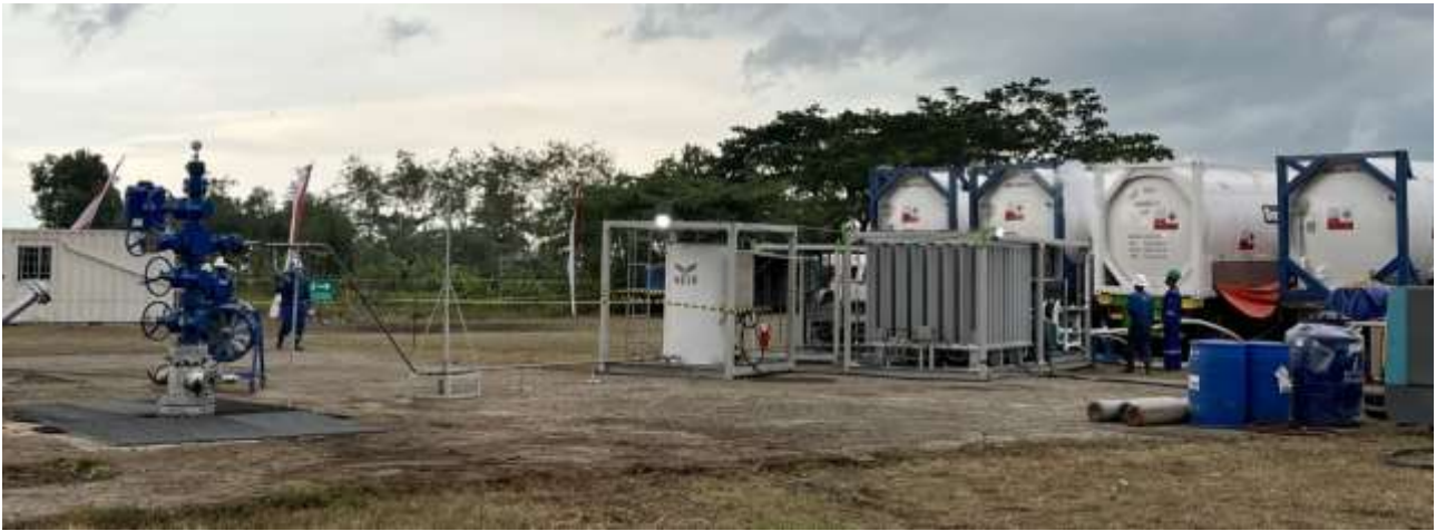
CO2 injection site at the Jatibarang oil field in West Java, Indonesia. White CO2 tanks are connected to the injection well shown on the left.
